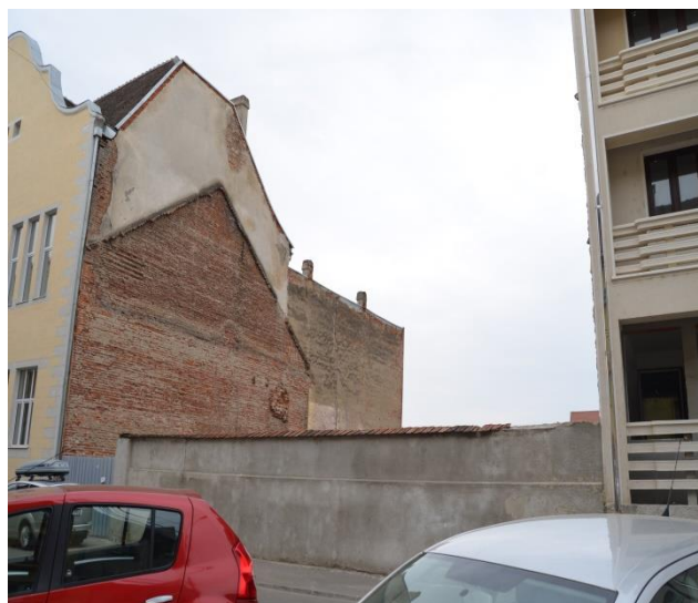
Figure 4 - Place of demolished house on Petőfi street
